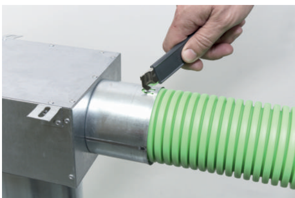
5) Press both locks to prevent the pipe from sliding out.
