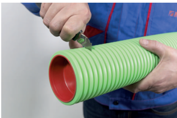
1) Cut the pipe to the required length at the groove in the corrugation.
